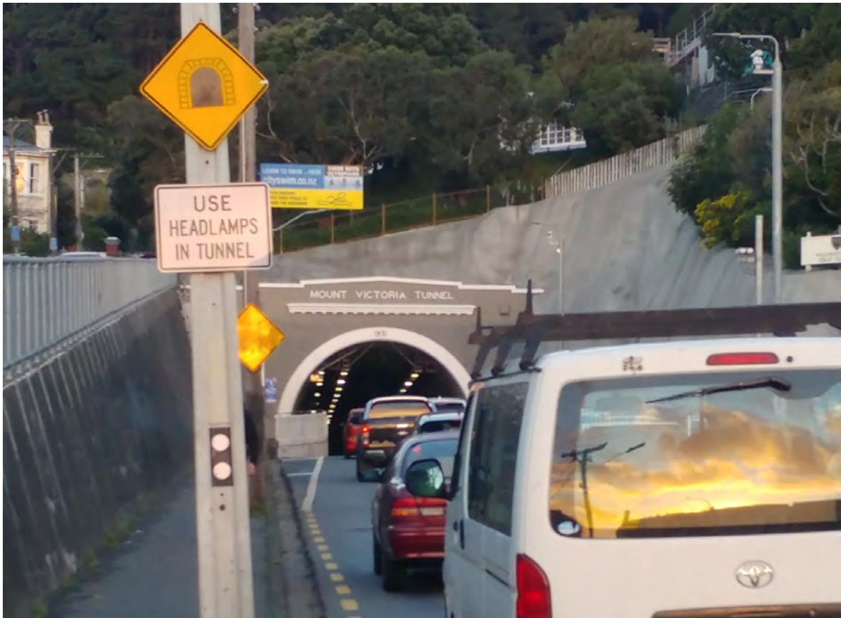
Mt. Victoria Tunnel. Wellington, New Zealand.
